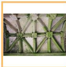
05 Porch groined ceiling.JPG
