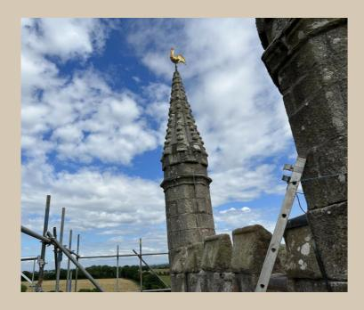
Phase 1 of the repairs to the church is complete. This was the grouting, repointing and re-roofing of the tower. We hope that it will now dry out over the coming years.
